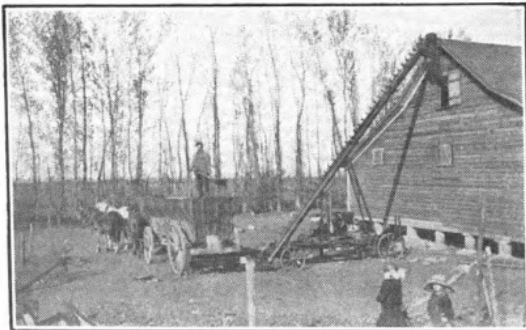
Portable Elevator Loading from Grain Tank to Elevator, Emil Lambert Farm
