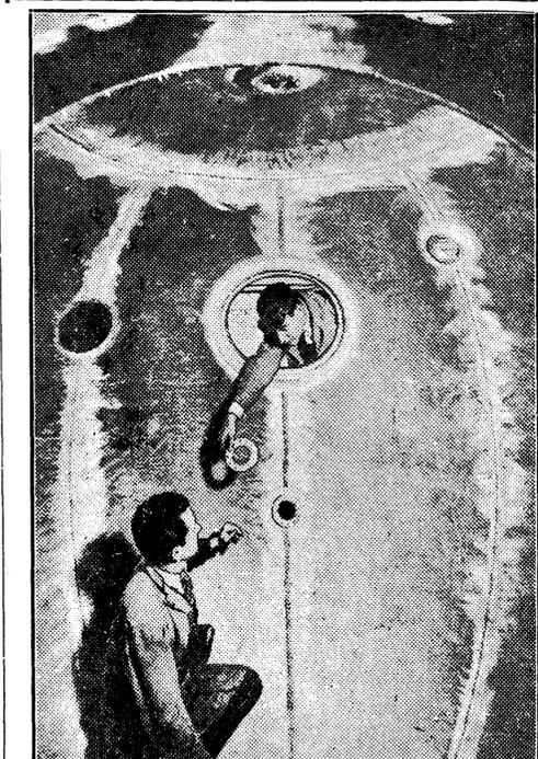
Taken through a manhole, this picture shows the inside of the huge metal ball in which Major William E. Kepner and Captain Albert W. Stevens of the U. S. Army will be sealed when they make their projected flight into the stratosphere this summer. The balloon and gondola are being constructed at Akron, Ohio.
